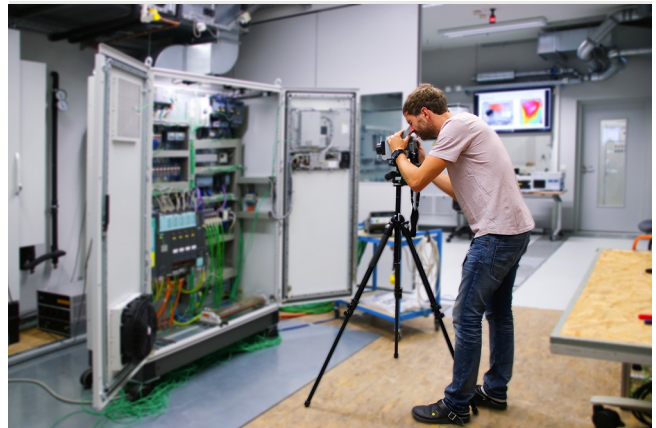
WKC - Test laboratory - Heat measurement
