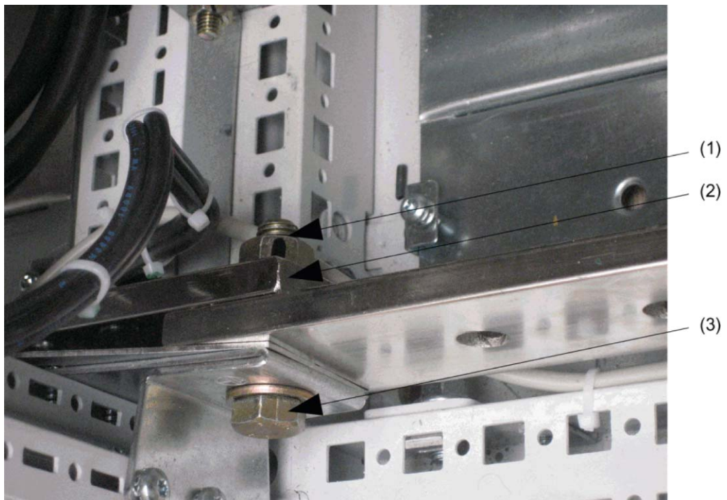
Figure 4-1 Connecting the PE busbar when cabinet units are installed side-by-side
