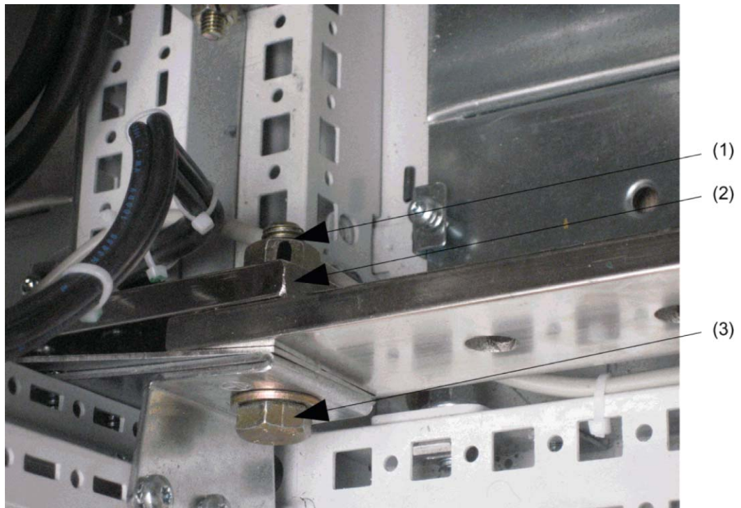
Figure 4-2 Connecting the PE busbar when cabinet units are installed side-by-side
