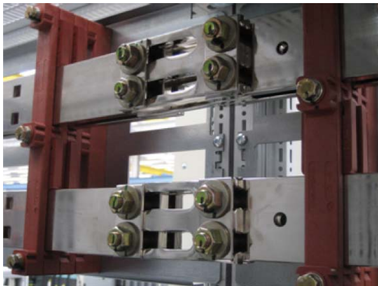
Figure 8-54 M80 - M87, DC busbar
