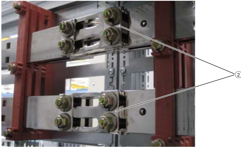
Figure 4-4 Connecting the DC busbar when cabinet units are installed side-by-side
