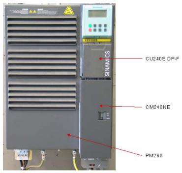
Figure 3-1 Chemical industry inverter (example)
