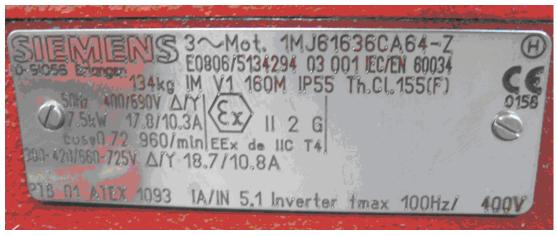
Figure A-2 Rating plate of an explosion-protected motor for inverter operation
