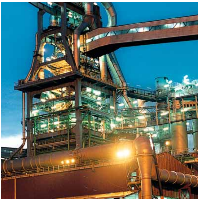
Industrial application: Refinery
