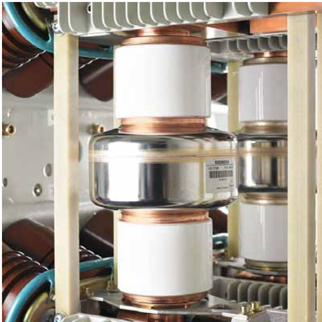
Vacuum interrupter
