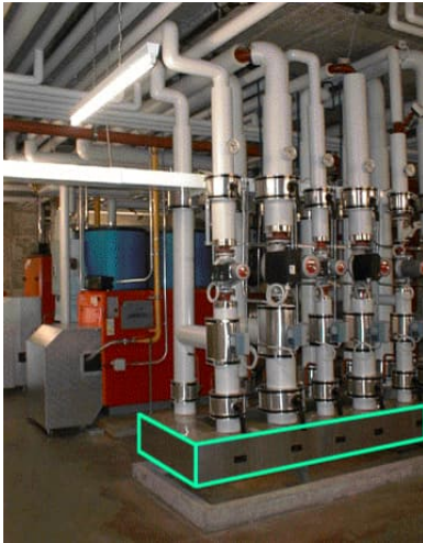
Distributor as the connecting element between heating generation and consumer side
