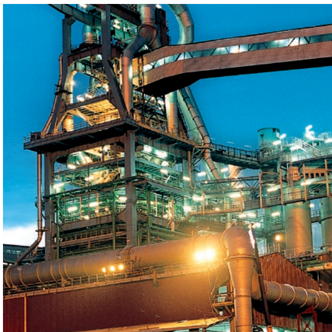
Industrial application: Refinery
