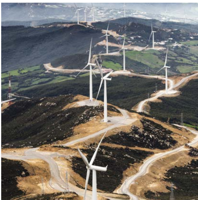
Wind power plant
