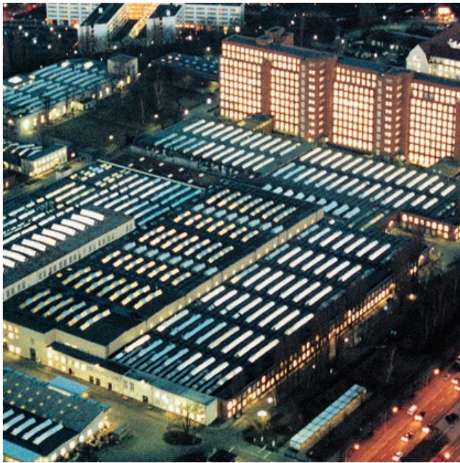
Switchgear Factory Berlin, Germany
