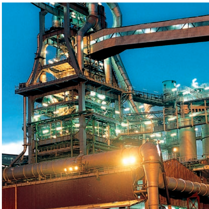
Industrial application: Refinery
