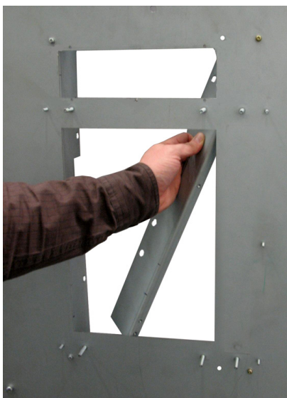
Locate the reinforcement plate on the mounting panel.
