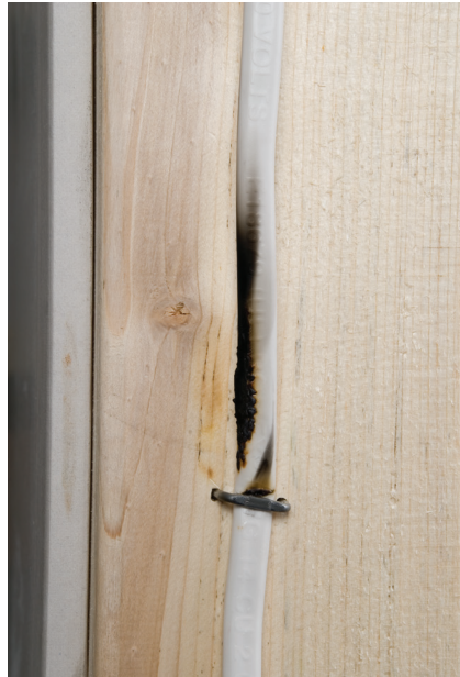
Damaged wiring
