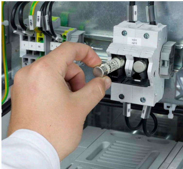
Figure 9-5 Replacing a cartridge fuse
