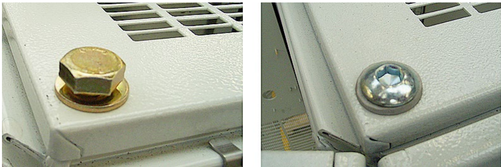
Figure 3-11 Delivery state (left), original roof screws (right)
