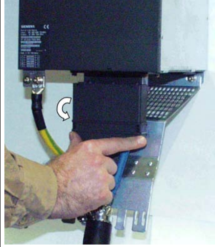
Close the cover of the terminal block.
