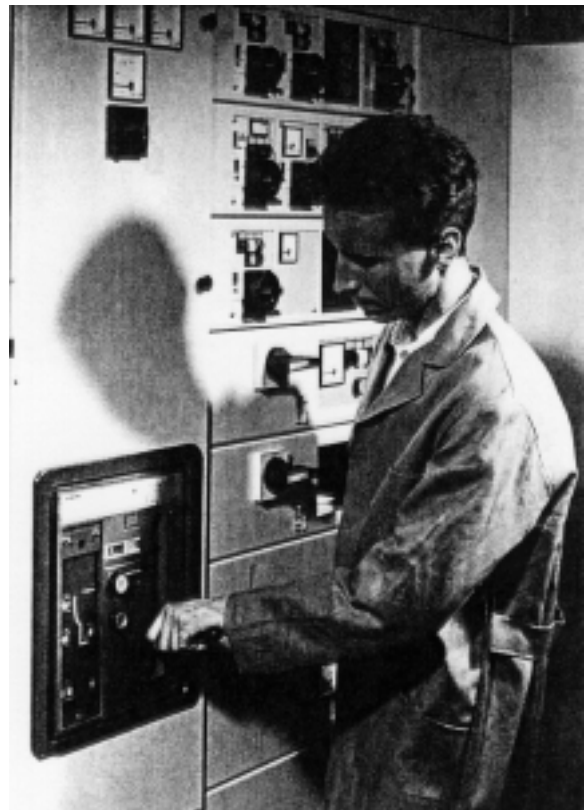
Fig. 1/1 3WN6 in a switchgear installation
