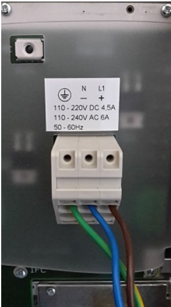
Figure 4-1 Connection of the supply voltage
